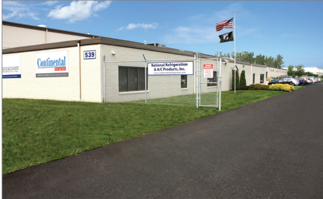
539 DUNKSFERRY ROAD, BENSALEM, PA, USA
